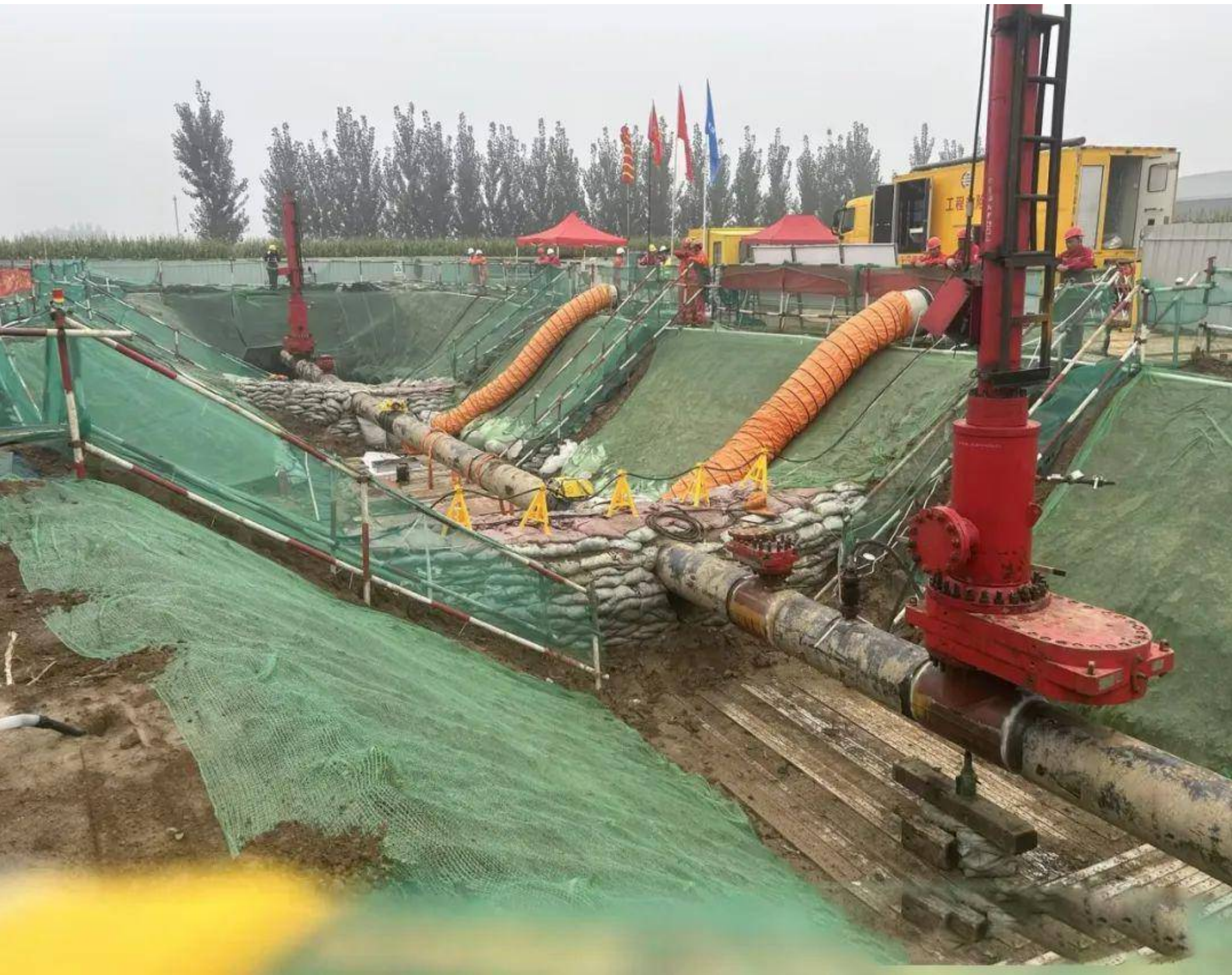
20" crude oil pipeline line stop
