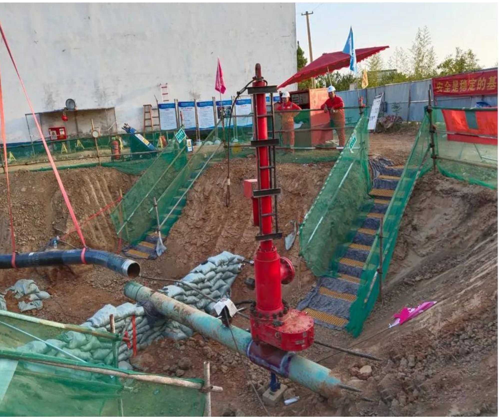
12" oil pipeline single line stop
