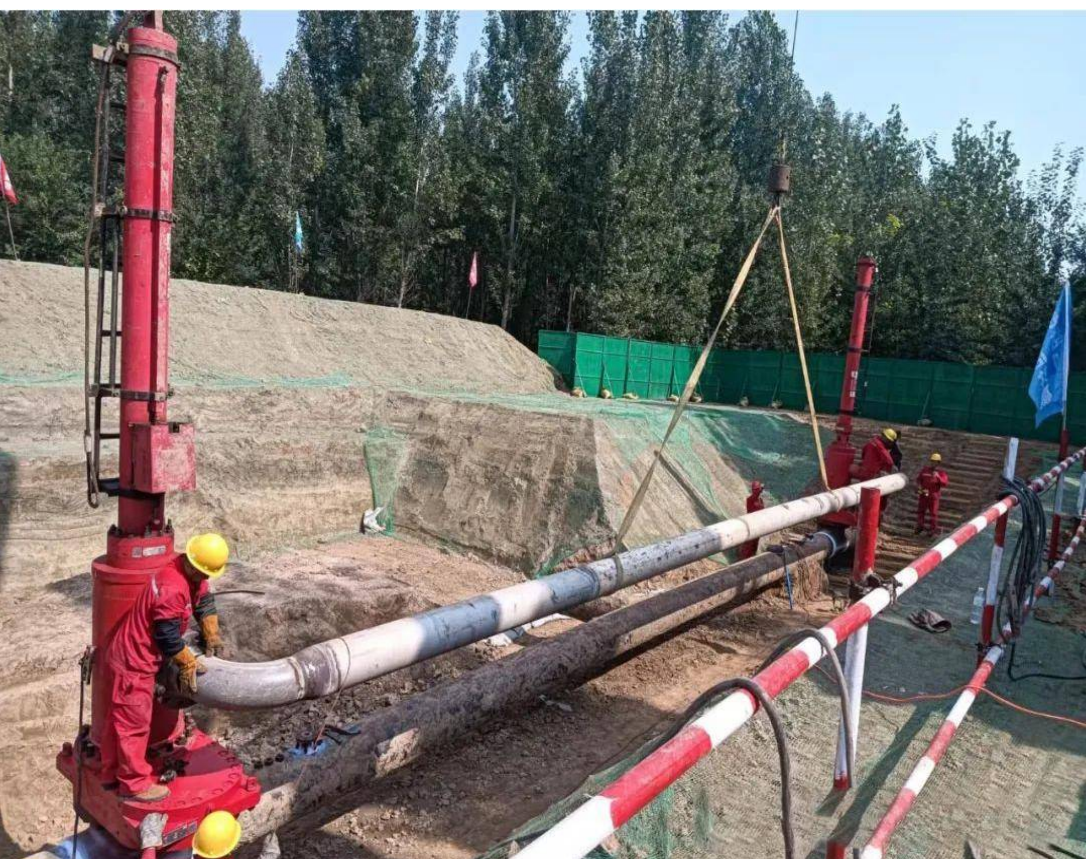
20" pipeline line stop
